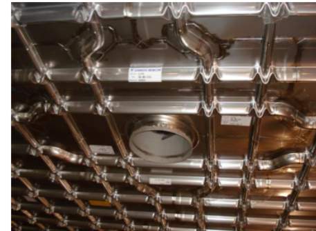
Roof nozzle penetration
