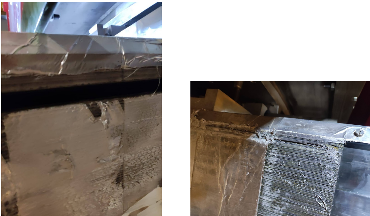
Figure 1.58: Delaminated ECAL modules.
