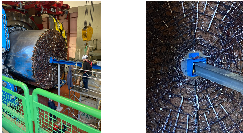
Figure 1.46: Left: extraction of the drift chamber at LNF. Right: zoom on the HEA200 beam and the trolley (detail in the text).
