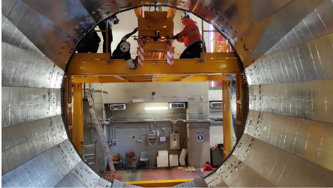
Positioning and precise aligning of extraction machine
