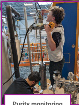
Purity monitoring installation
