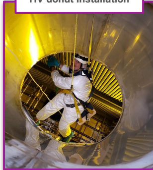
HV donut installation
