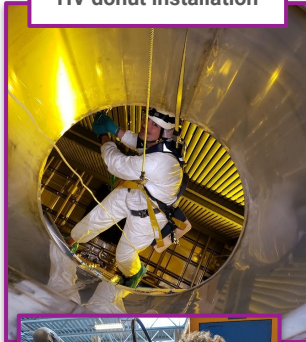
HV donut installation
