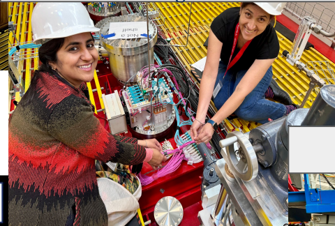
Towards commissioning: Installing cables
