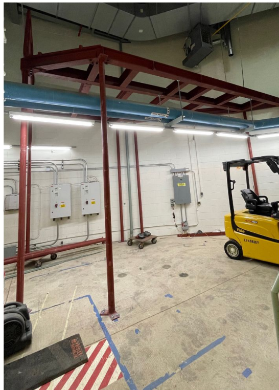
Construction started in 2023.
