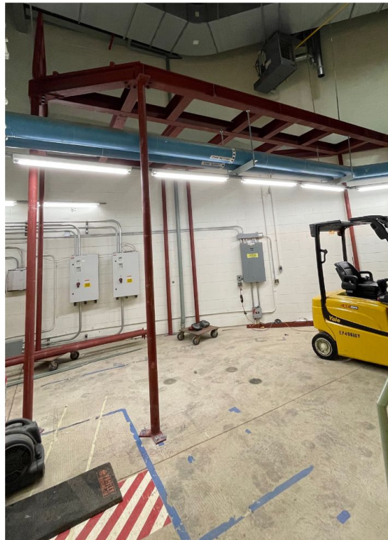
Construction started in 2023.
