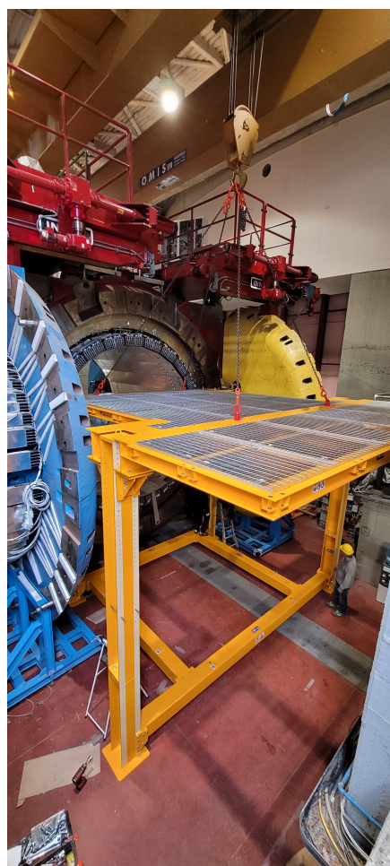
Figure 1.6: Movable platform for barrel modules extraction at LNF.
