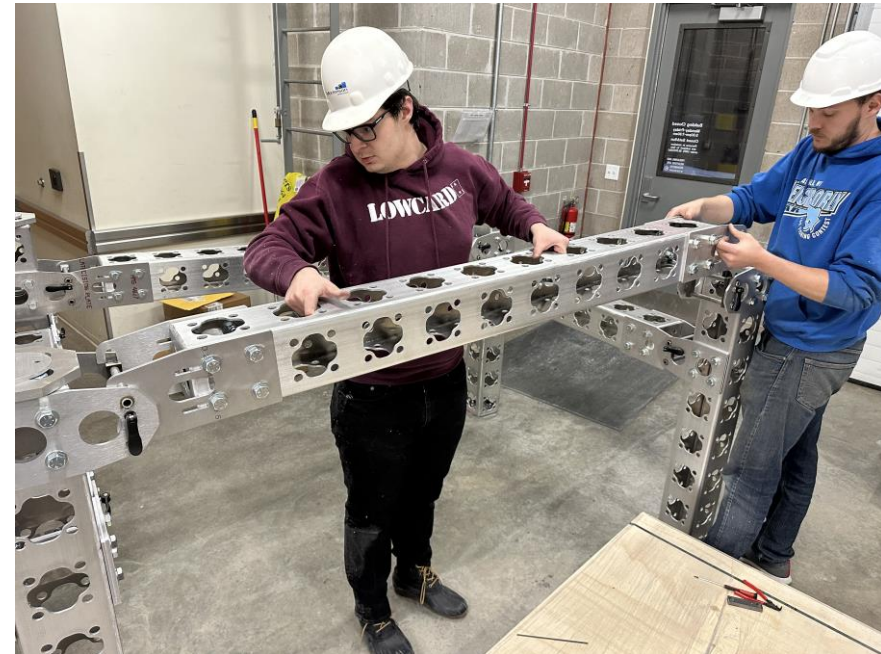
2) Spotters Disassemble the Truss
