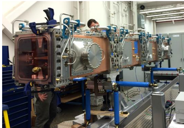
Water cooling system installation
