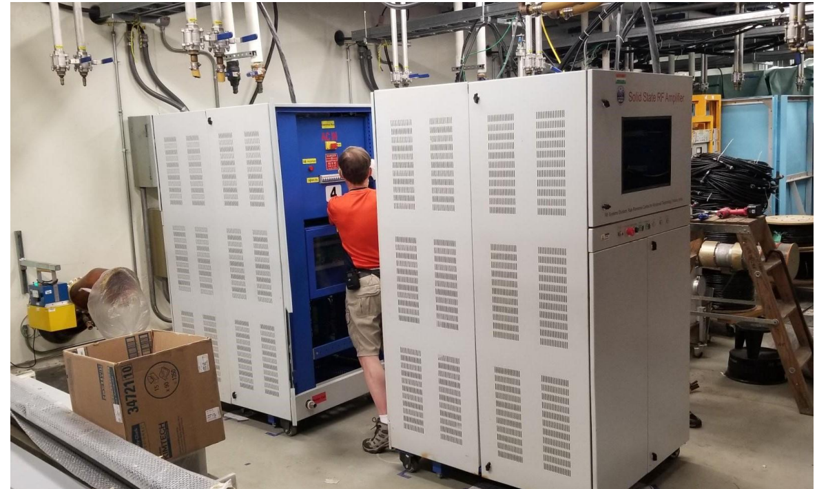
RRCAT 40 kW 650 MHz prototype amplifier just arrived, being assembled, in preparation for testing
