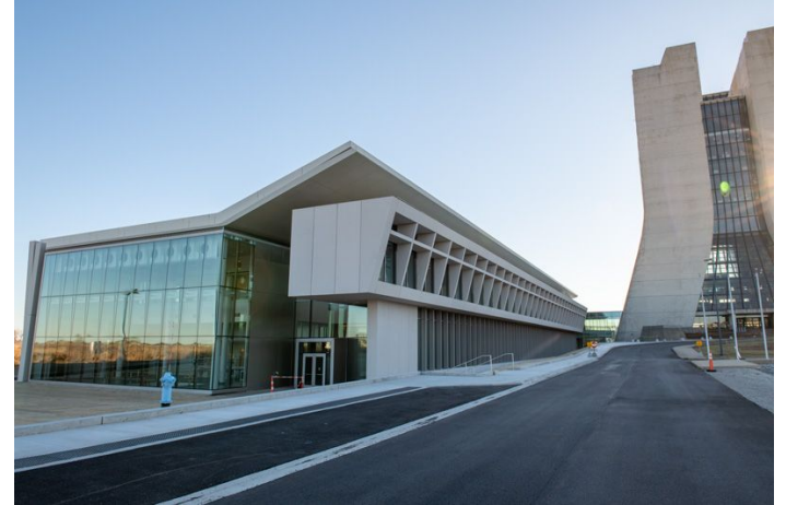
Interior and exterior of IERC
