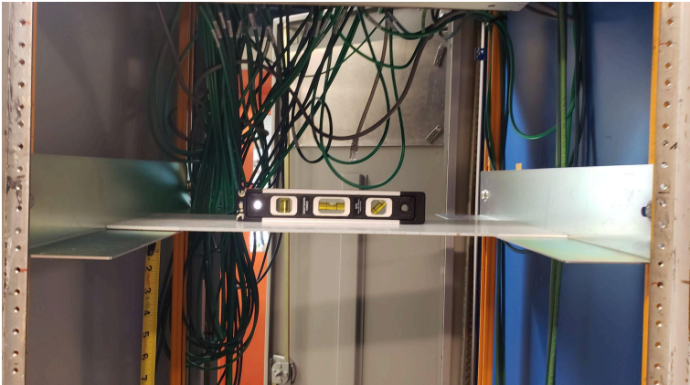
Figure 8. Spirit level used to ensure correct leveling of shelf
