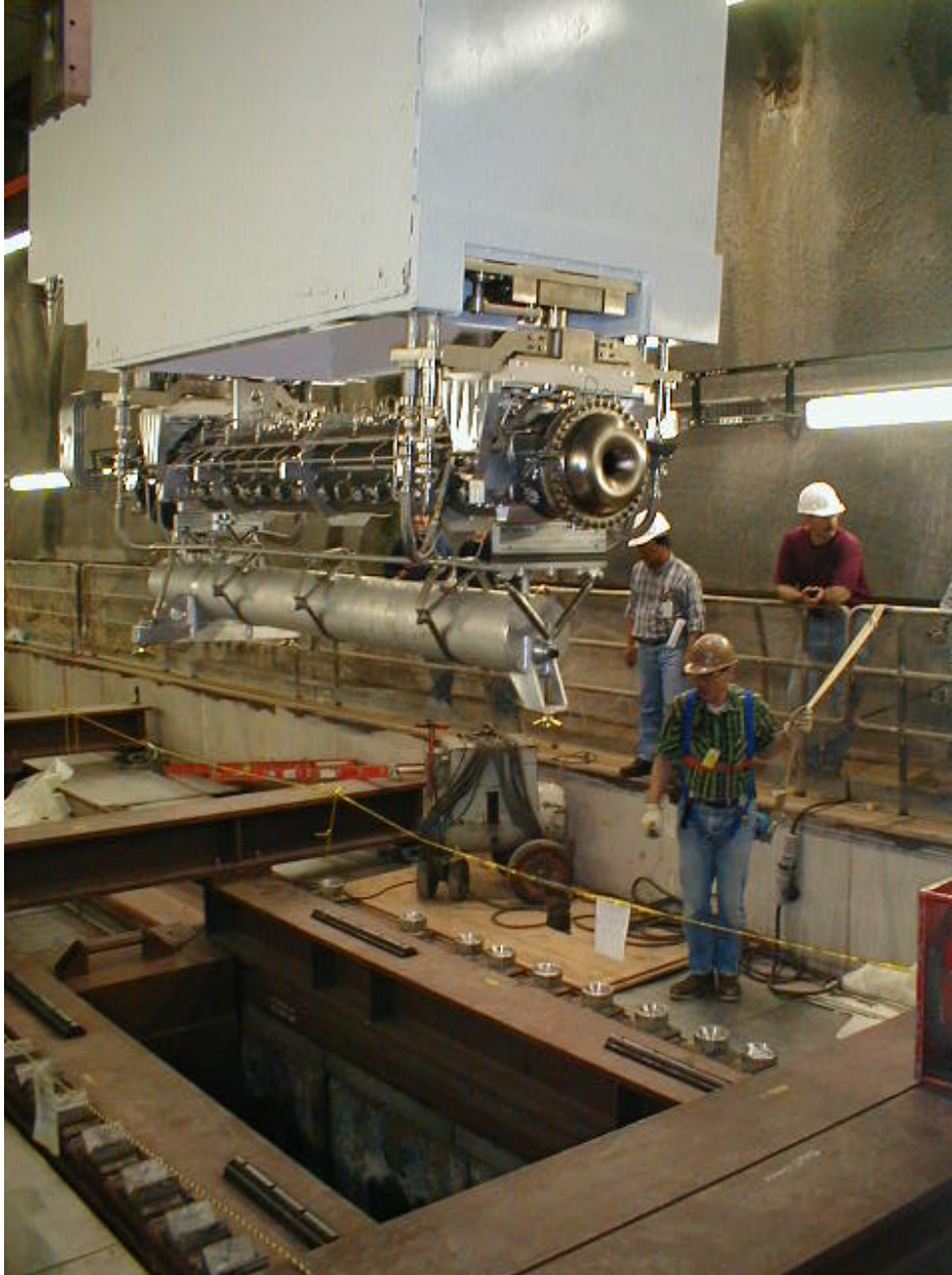
Figure 21. NuMI Horn 1 and positioning module installation in beamline chase.
