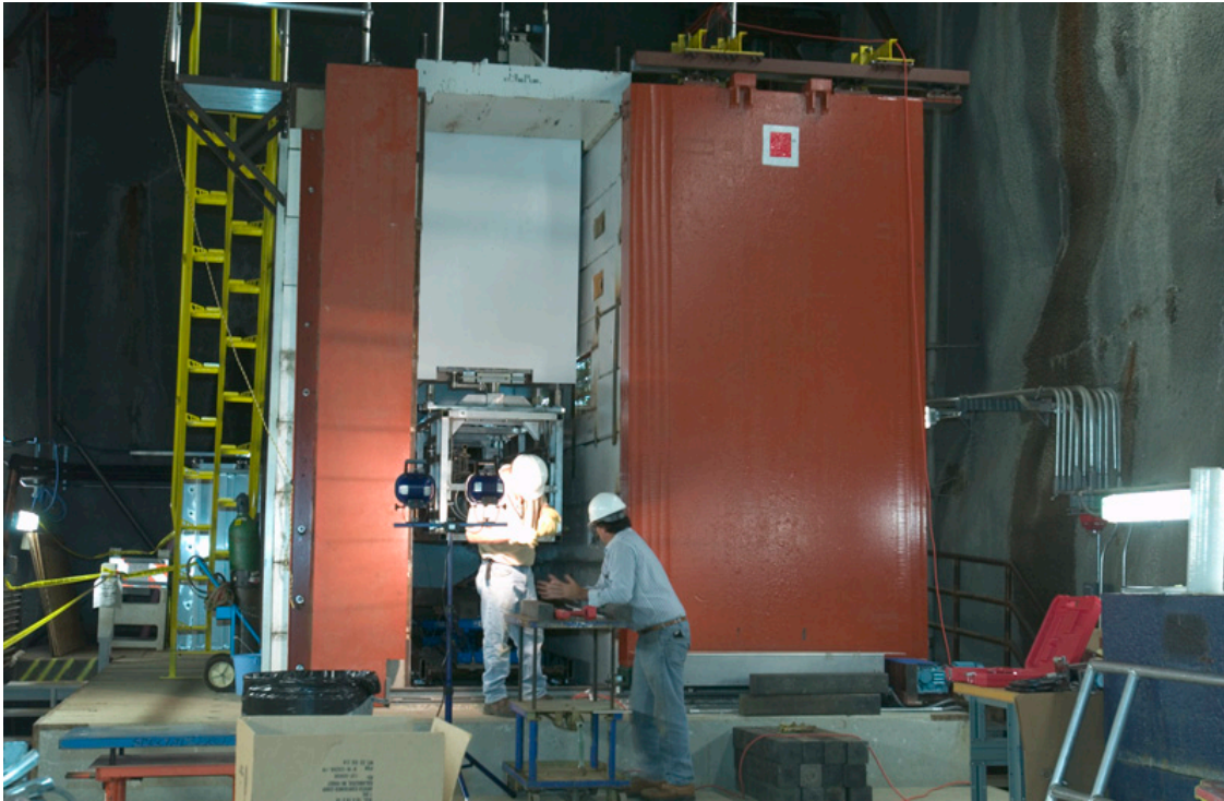
Figure 10. NuMI Workcell for hot handling operations and failed component replacement. Image shows NuMI target module in the workcell for a hot handling procedure dry run during NuMI construction
