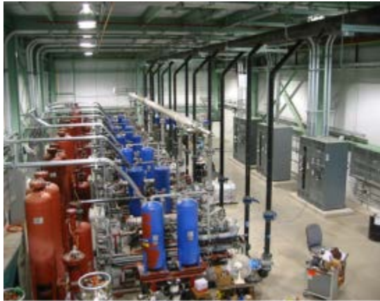
Reused TeV compressors for CMTF
