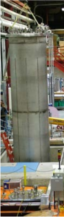
VTS3 being installed
