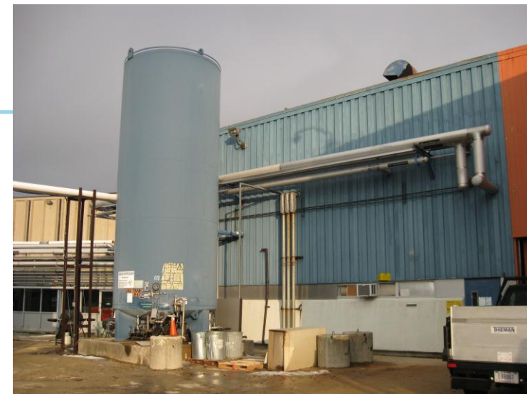
IB1 LN2 dewar and transfer lines
