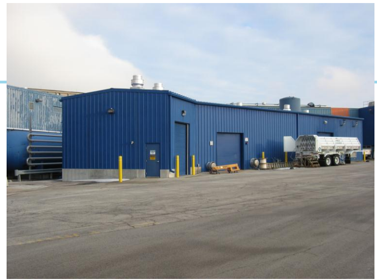
IB1A, extension, and GHe tube trailer
