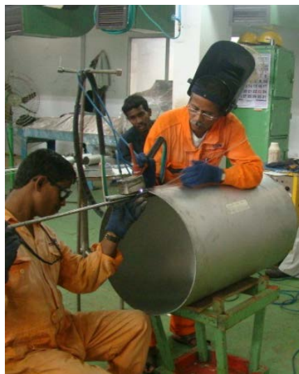
Preparation for Welding (back purging and trailing shield arrangement)
