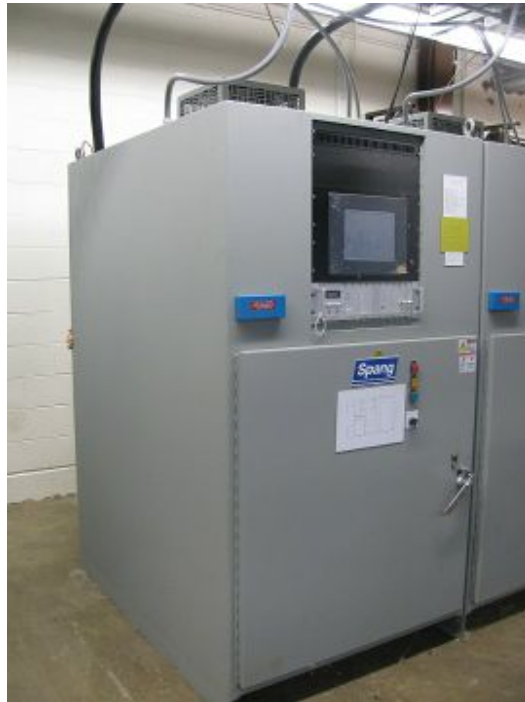
Figure 4.90. Example of an SCR type Power Supply.
