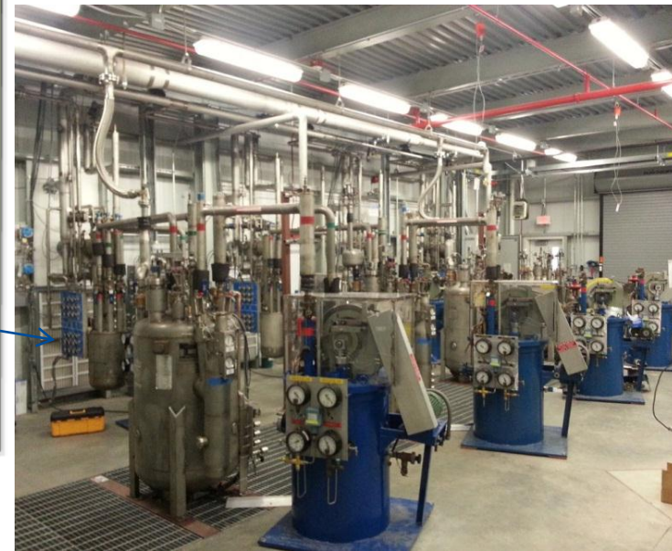
Much of cryo equipment refurbished / reengineered Tevatron equipment
