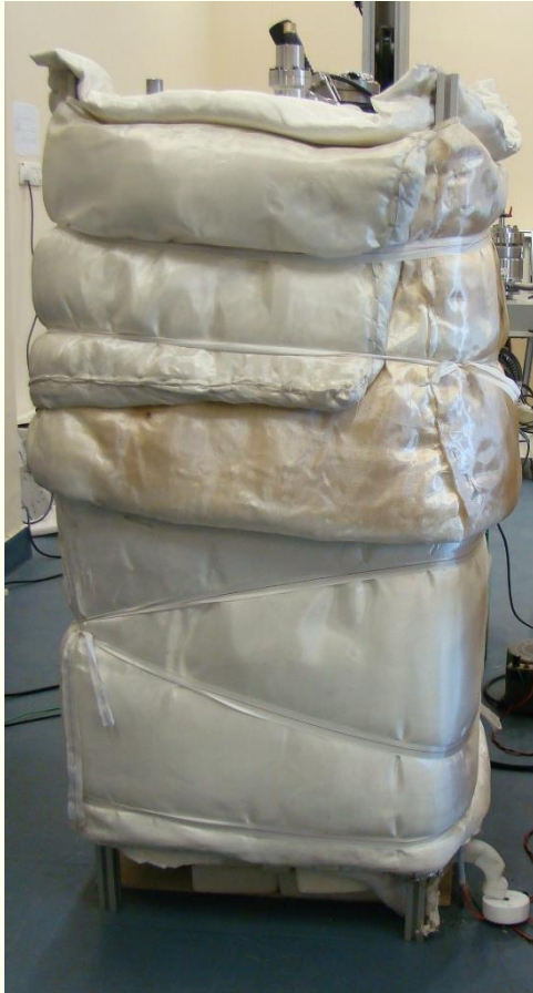
Low temperature baking facility for 650 MHz
