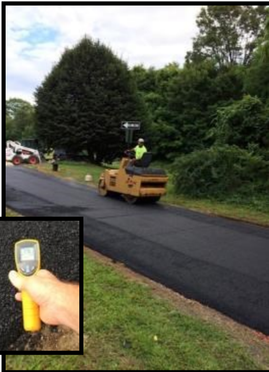
Paving with 113°C (236°F) asphalt at Centerdale School in Providence, RI
