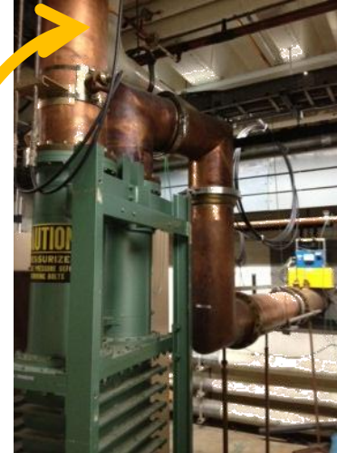
FNAL/Linac 200 MHz coax line ( \cong 40ft long)
