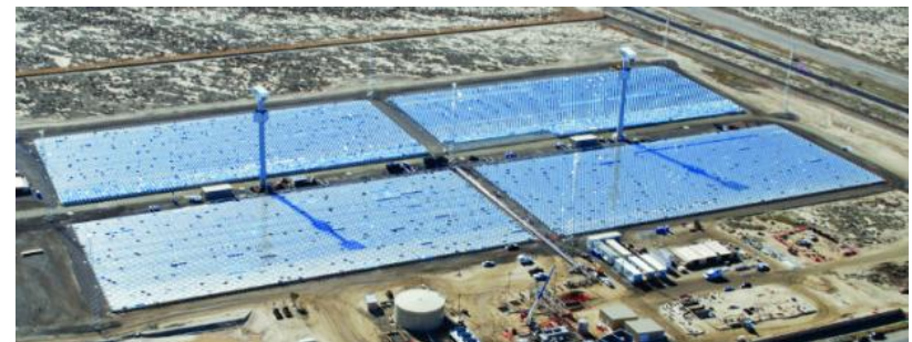
eSolar array in southern California
