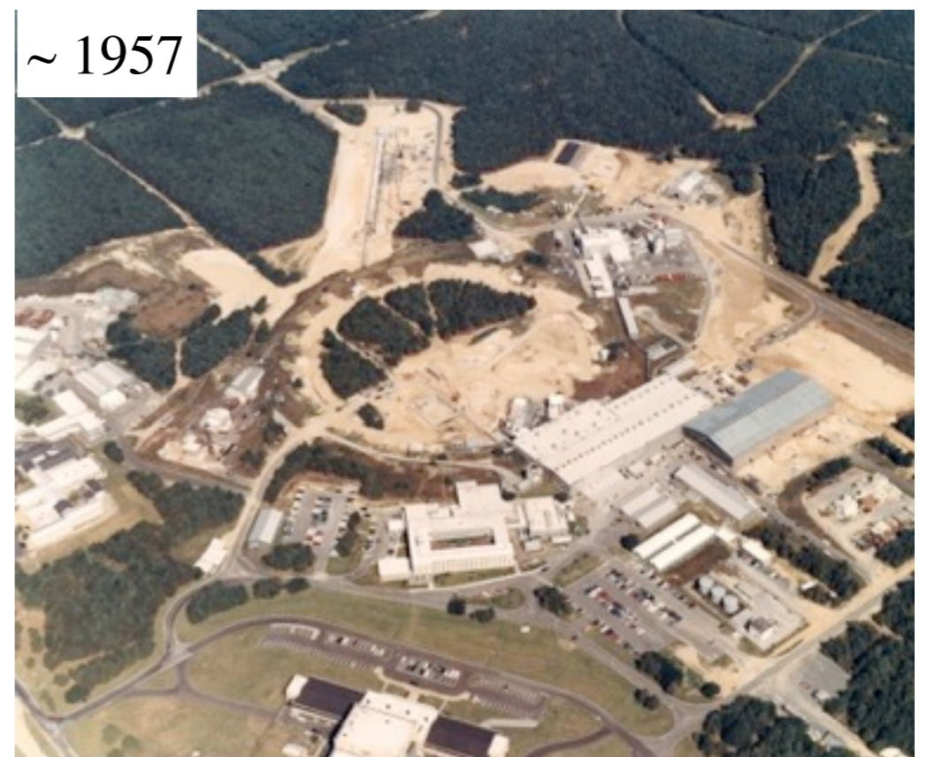
AGS construction, Brookhaven, New York
