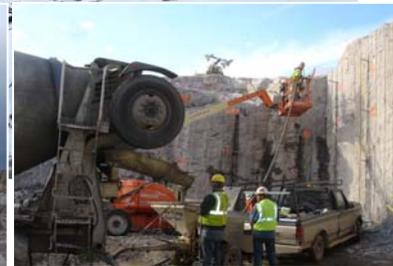
Rock bolts installed in all walls of first lift
