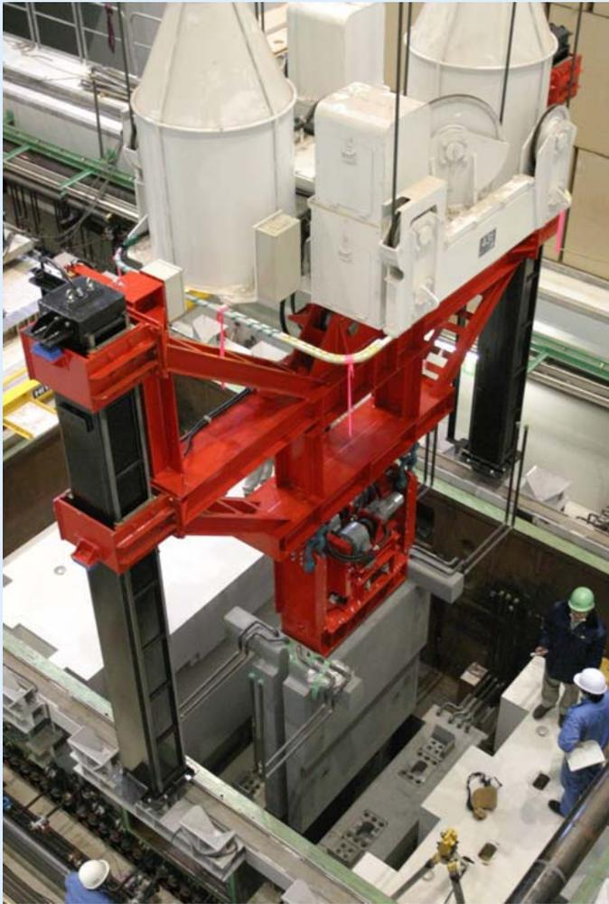
2.2m thick iron shields remotely installed
